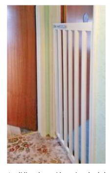
A sliding bar with spring loaded plunger that secured it in position provided the locking mechanism. It was designed so that the boy was unable to see it and unlock it.
