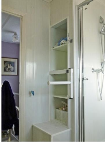
The rectangular section steel mounting included a series of attachment holes to allow the rail to be height adjustable. All steel work was powder-coated white and plastic end caps fitted to the RHS.
