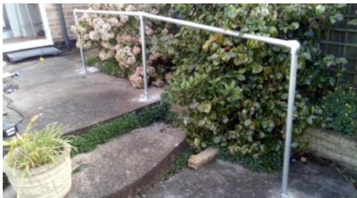
An elderly Burton man with walking problems was struggling to reach his lower garden. A handrail on some steps to the lower part of his garden was needed to aid his stability. The path was surveyed and several handrail parts were purchased. The rail was assembled on site and provides a safe and secure means of getting down to the garden.
