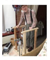
Two handrails were made so he can hold one with his right hand as he faces outwards leaving his room and another as he returns in the opposite direction. They are fixed to a platform which in turn is screwed to the floor through the grout so as not to damage his expensive floor tiles.
