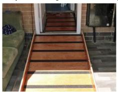
together by steel hooks locked in place by threaded turn-wheels. The slope is 1 in 12 and the ramps are finished in matt varnish with antislip strips placed laterally at intervals.
